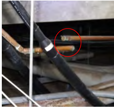
Broken leaking pipe (break circled in red)
