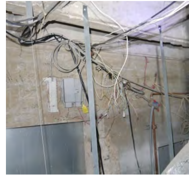
Exposed low voltage wires
