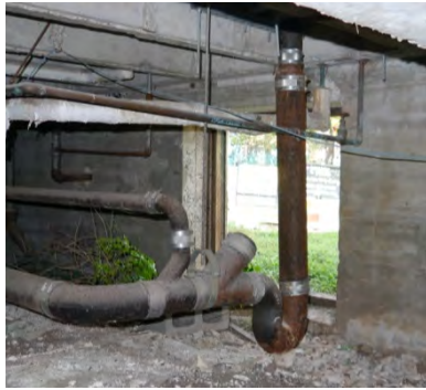
Degraded insulated & corrugated pipes
